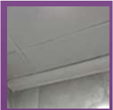
CEILING ( PVC PANNEL )
